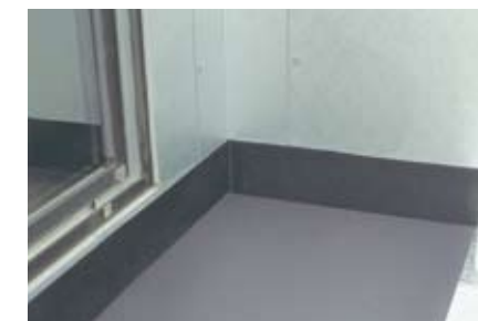
Kolpak freezer floor panels exceed R-28 insulation rating
